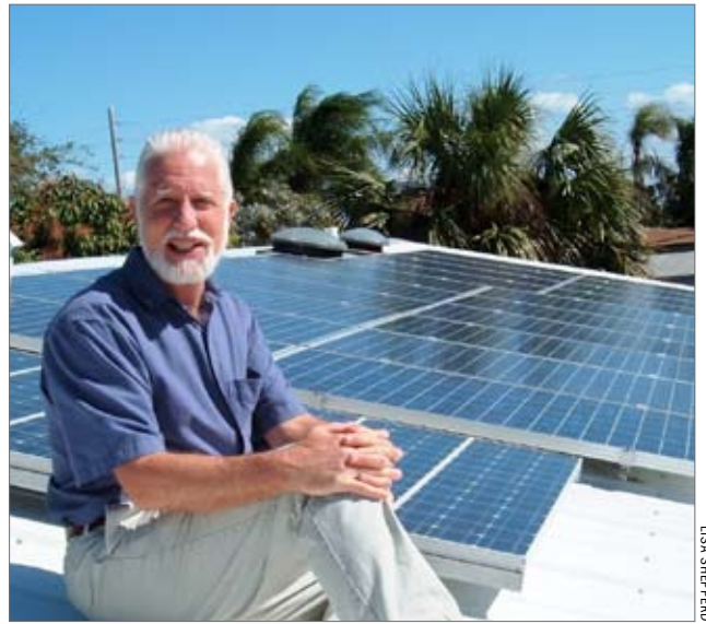
Danny Parker sits on the roof of his remodeled home with white metal roof, solar hot water heater, and 4.92 kW PV system.
